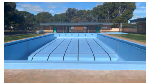
Main Swimming Pool Completed
