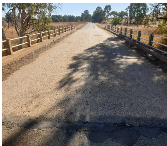
Forest Road Bridge 1 - Barrier
