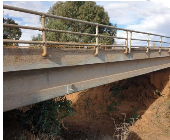
Figure 3.14 Appila-Tarcowie Road Bridge
