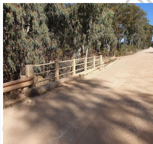
Forest Road Bridge 2
