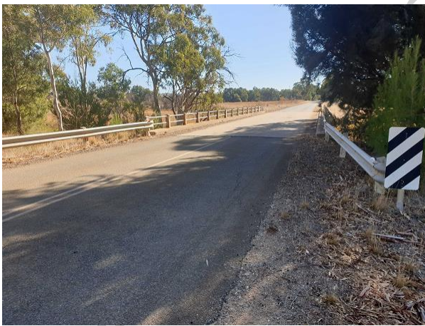
Figure 3.15 Forest Road Bridge 1
