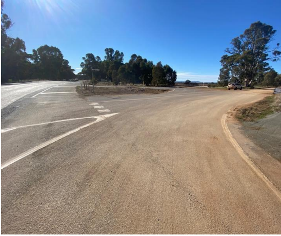
Rural Heavy Use Hotmix Bitumen Road
