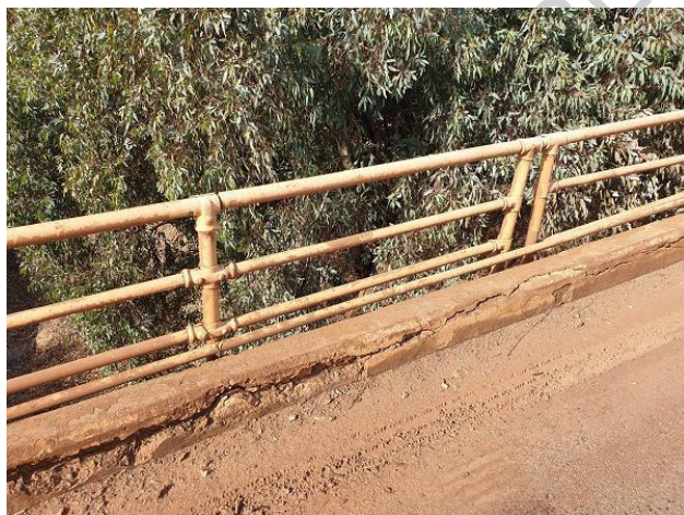
Appila Tarcowie Road Bridge
