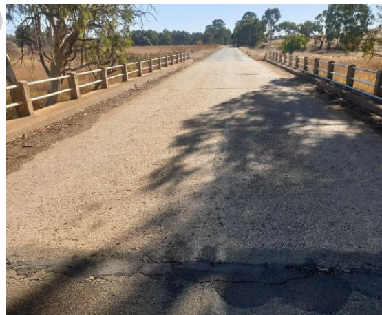
Figure 3.16 Forest Road Bridge 1
