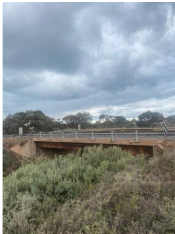
Figure 3.13 Port Germein Bridge
