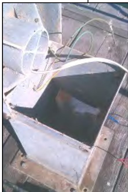
Picture left shows the base of the Jetty light where the solar battery is housed. The safety bolts have been drilled out and the light lowered. The electronic components that operate the light have been removed.
