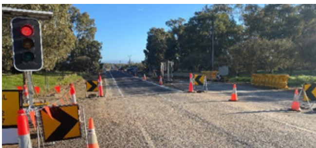
Spring Creek Bridge Upgrade
