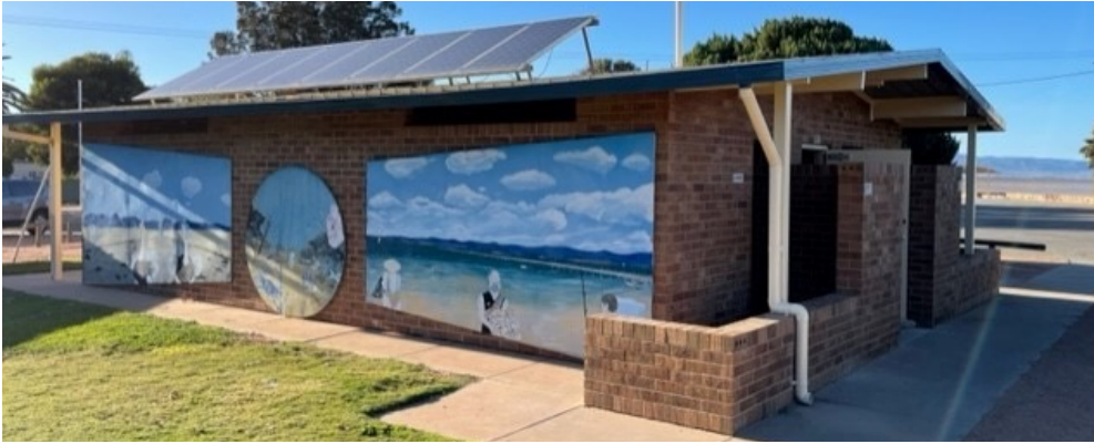
Port Germein Toilet Block
