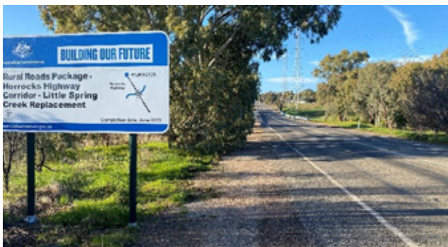
Little Spring Creek Upgrade
