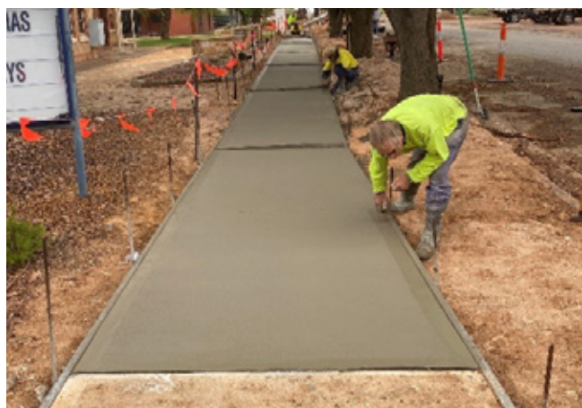
Construction of new concrete path on Stephens Street in-front of school
