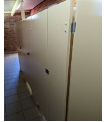
Port Germein Toilet Block
