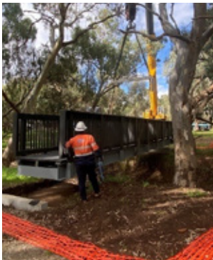
Max Cranes placing bridge at Wongabirrie Park in Wirrabara and Rocky River at Stone Hut.
