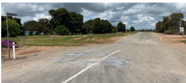
Patching Dunston Road, Booleroo Centre
