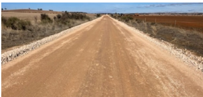
Collins Road completed
