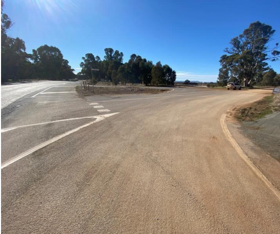
Rural Heavy Use Hotmix Bitumen Road
