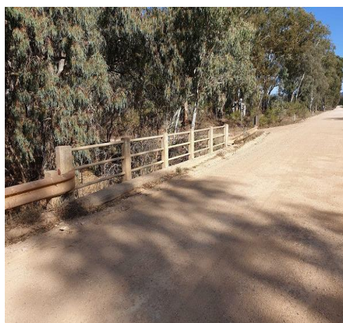
Forest Road Bridge 2
