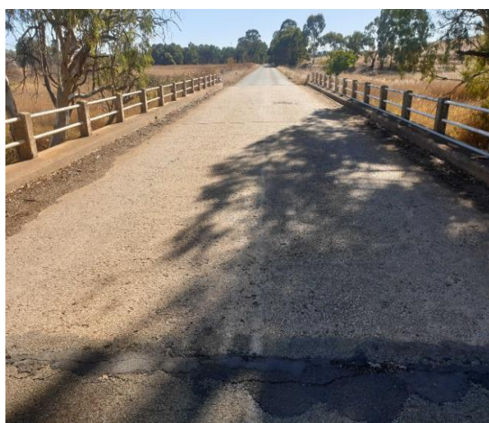
Forest Road Bridge 1 - Barrier
