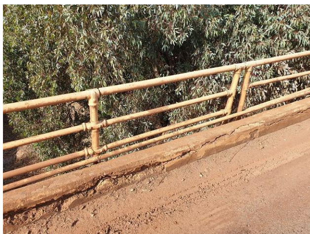
Appila Tarcowie Road Bridge
