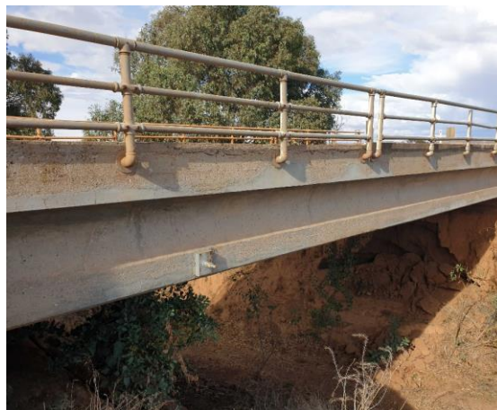
Figure 3.14 Appila-Tarcowie Road Bridge
