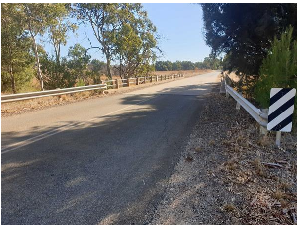
Figure 3.15 Forest Road Bridge 1
