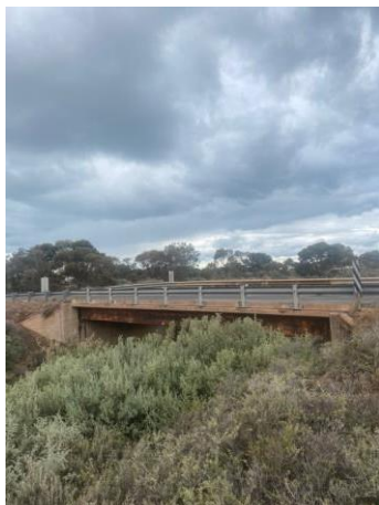
Figure 3.13 Port Germein Bridge
