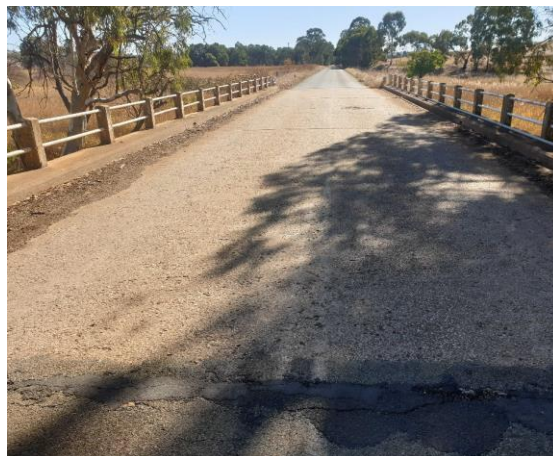
Figure 3.16 Forest Road Bridge 1
