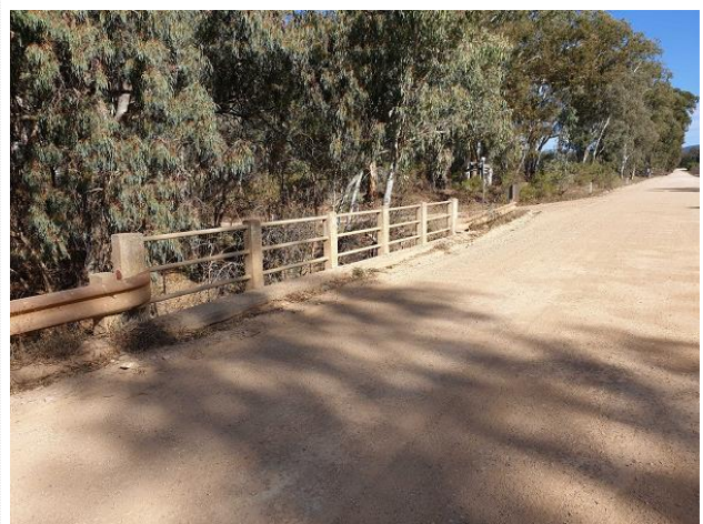
Figure 3.10 Forest Road Bridge 2
