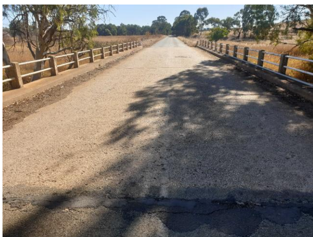
Figure 3.9 Forest Road Bridge 1 - Barrier
