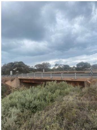
Figure 3.13 Port Germein Bridge
