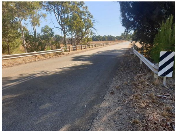
Figure 3.15 Forest Road Bridge 1
