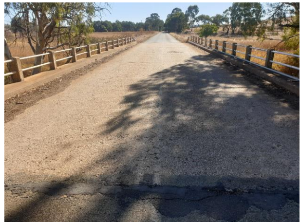
Figure 3.16 Forest Road Bridge 1
