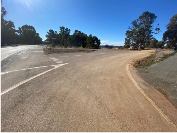
Rural Heavy Use Hotmix Bitumen Road
